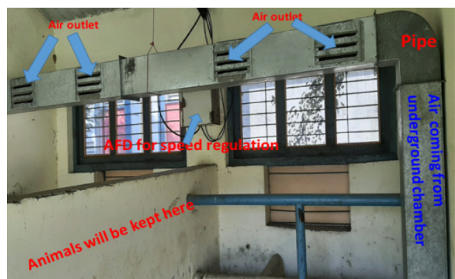
Fig. 2: Major components of geothermal system (Inside view of animal shed)
